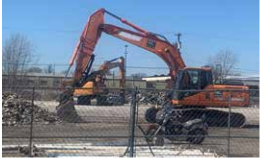
Excavators clear debris at the site of Afena Federal Credit Union's new corporate headquarters.
